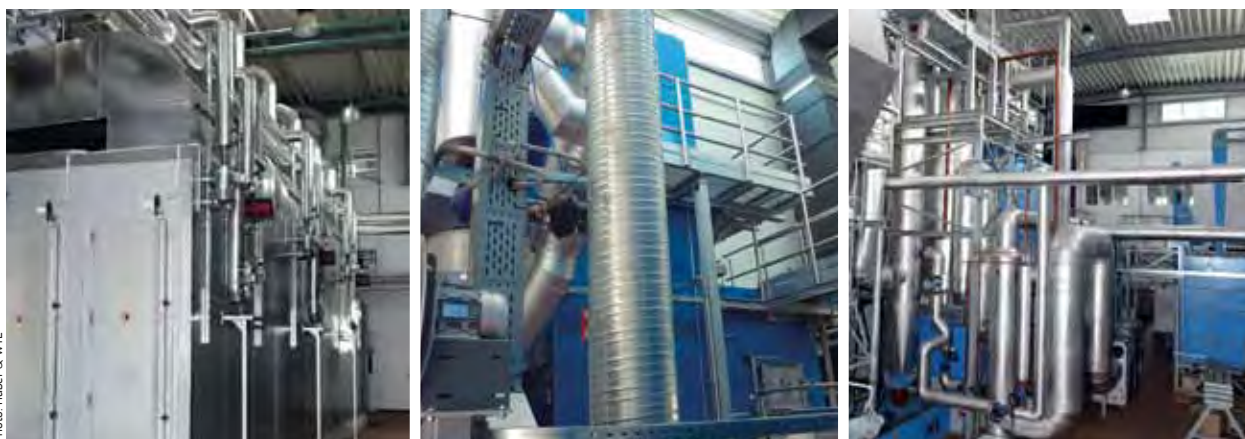
Power created from drying an initial batch of sludge can be used to dry subsequent batches in a closed-loop system
